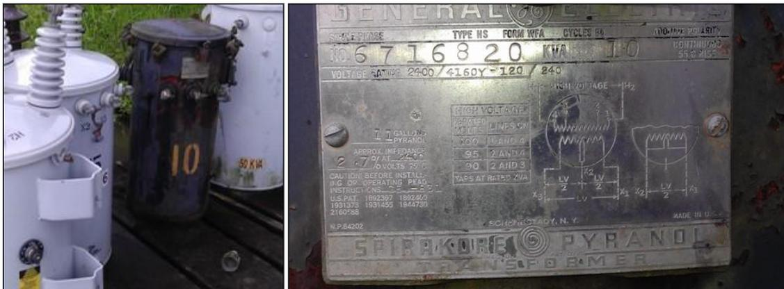
**Figure 2.10 – Filled Distribution Transformers including one containing Pyranol**
