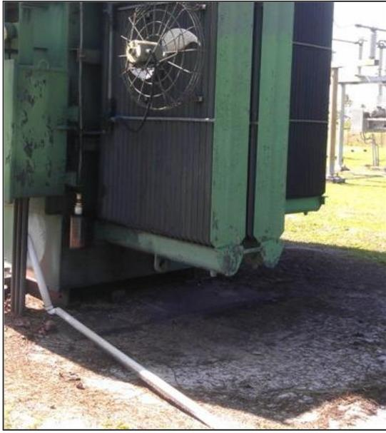
**Figure 2.18 Contamination over 50 ppm Around an Active Station Transformer - Canefield**
