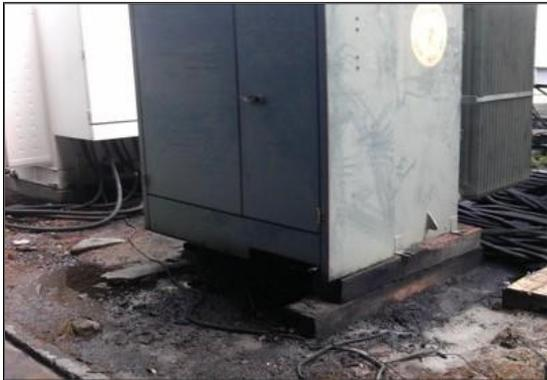
**Figure 2.20 Contamination over 50 ppm Around a Grounding Transformer - Versailles**
